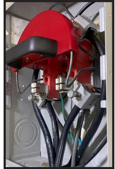
The AE Products Hot Jaw Safety Cover is a cost effective safety product for electrical workers if power disconnect is not an option. This non-conductive design allows work in the lower part of the meter can while blocking the upper jaw blades.
